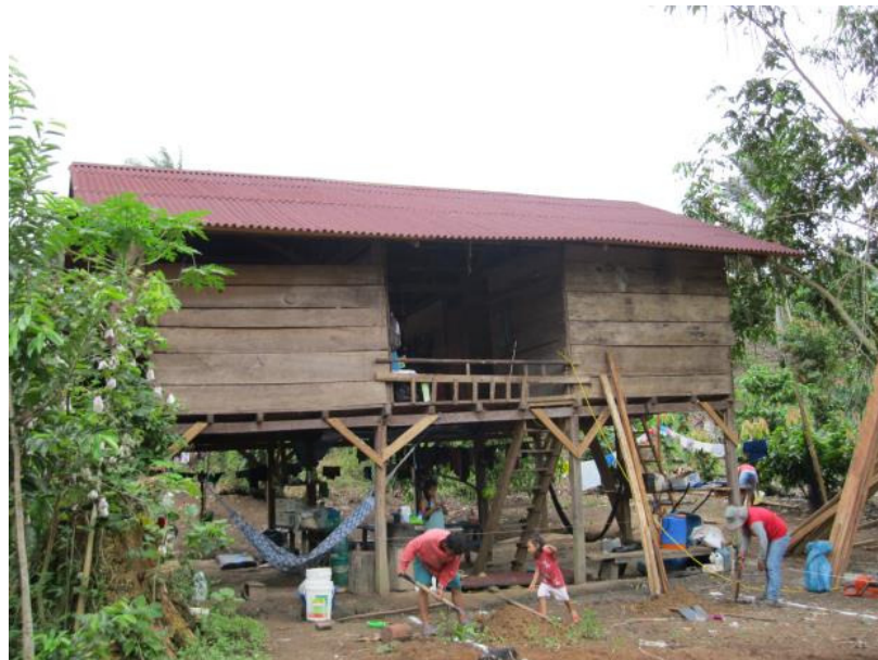
House with new roof.
