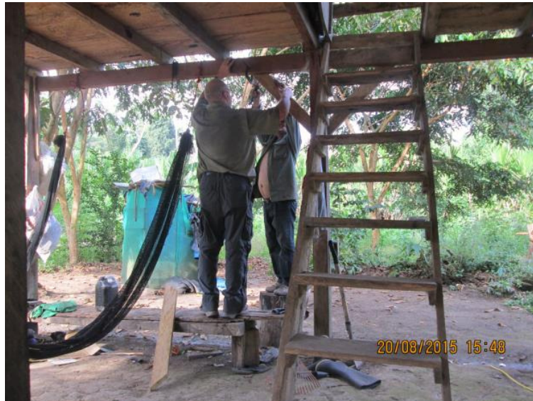
Arthur and Moises adding braces to structure.
