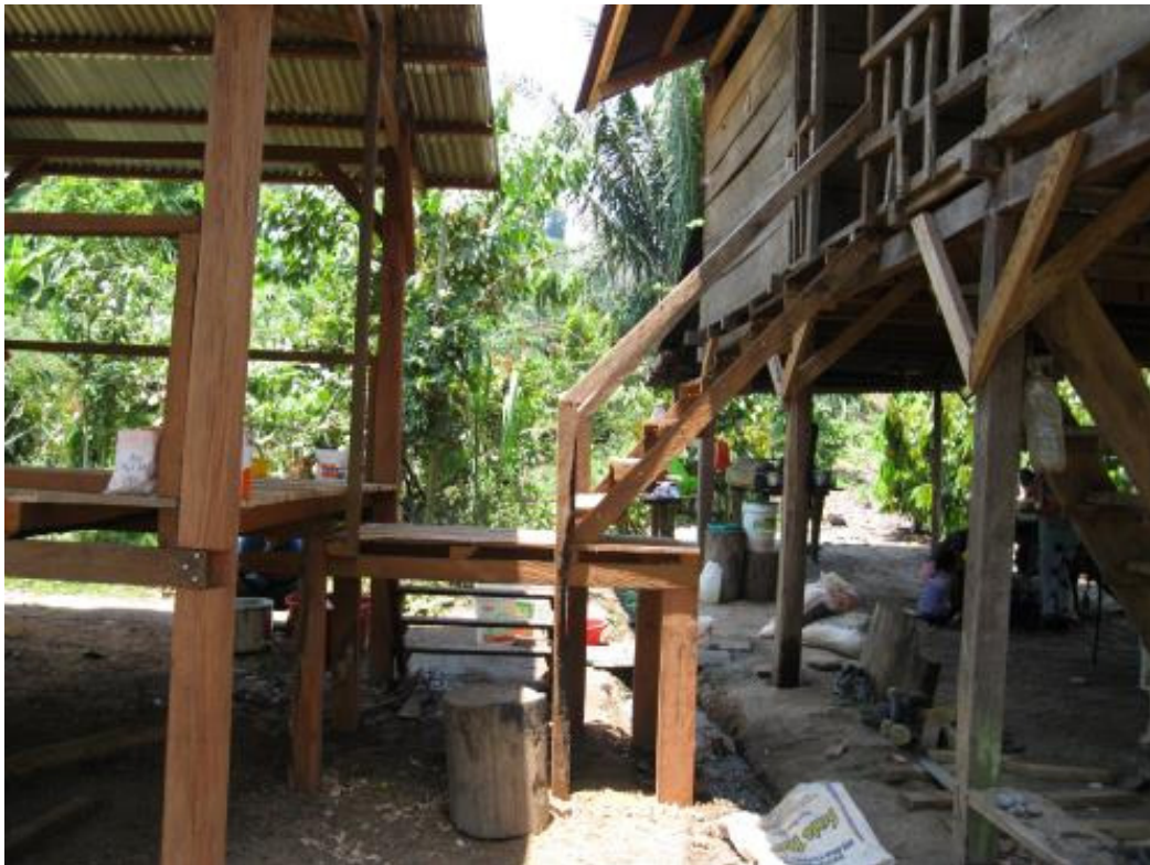
New stairs for dining area and house.
