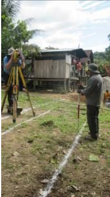
Arthur and Ivan setting elevations.
