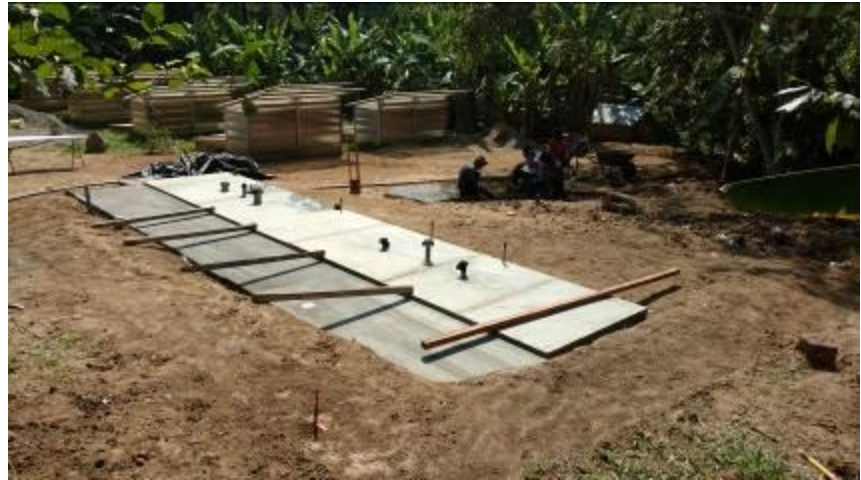
Finished bathroom floor and side walk.
