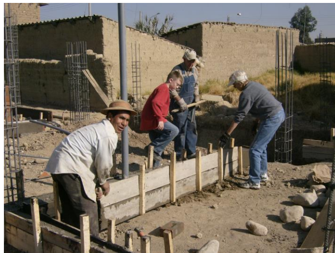
Constructing the sub-walls.
