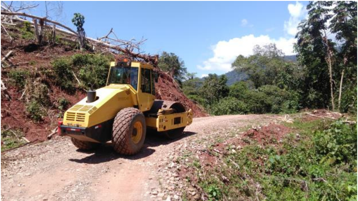
Road surface stabilization.
