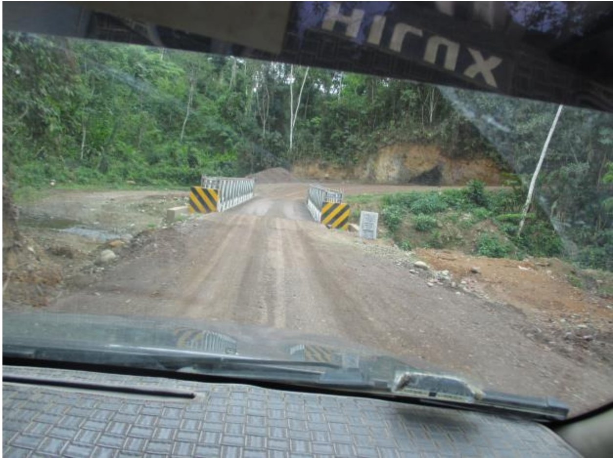
Typical road stabilization and new bridge.
