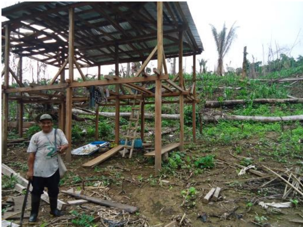
Construction of temporary structure at site with neighbor, Grimaldo Méndez.
