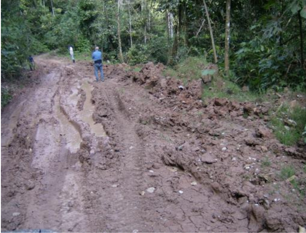
Typical road condition between Libertad de Anapati and project site.
