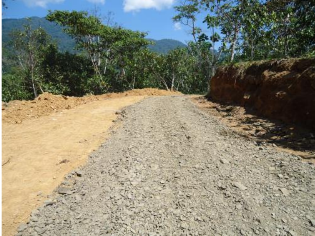
Road improvement work between Santa Cruz de Anapati and Libertad de Anapati.
