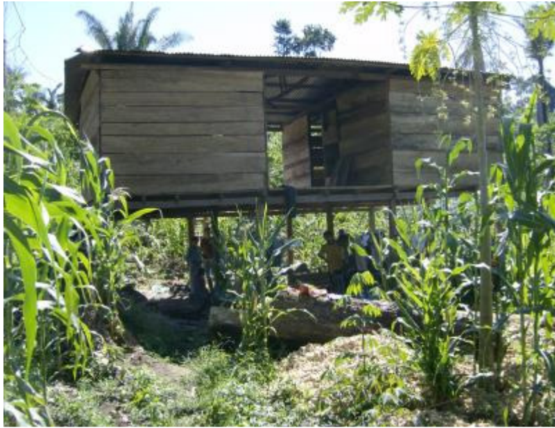
Temporary Structured completed.
