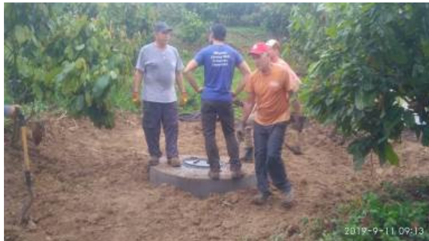
Concrete casing around water collection tank completed.
