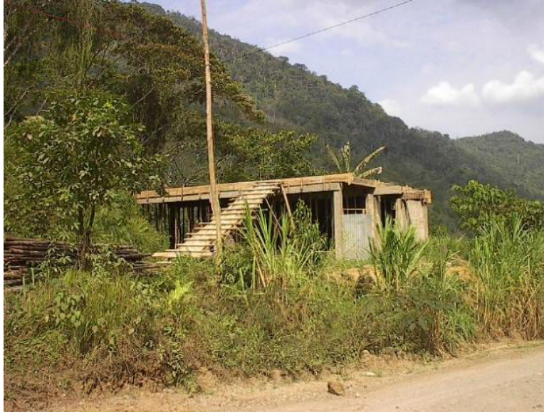
Church structure at Puente Paucartambo.
