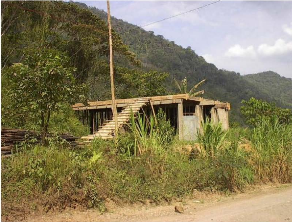
Church structure at Puente Paucartambo.
