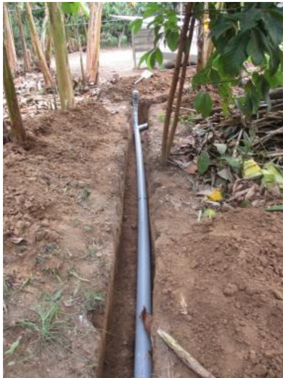
Drain piping installation.
