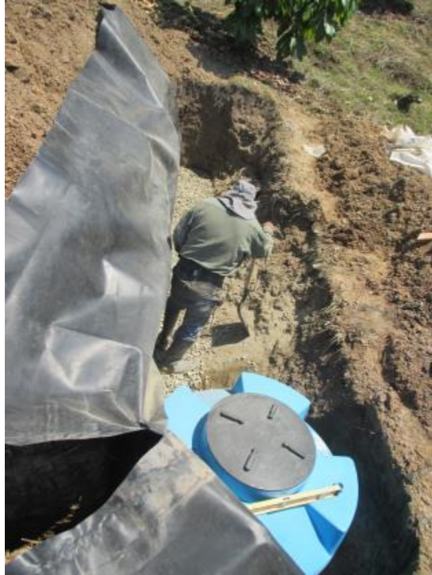
Installation of tank, cutoff membrane, and one of the collector lines.
