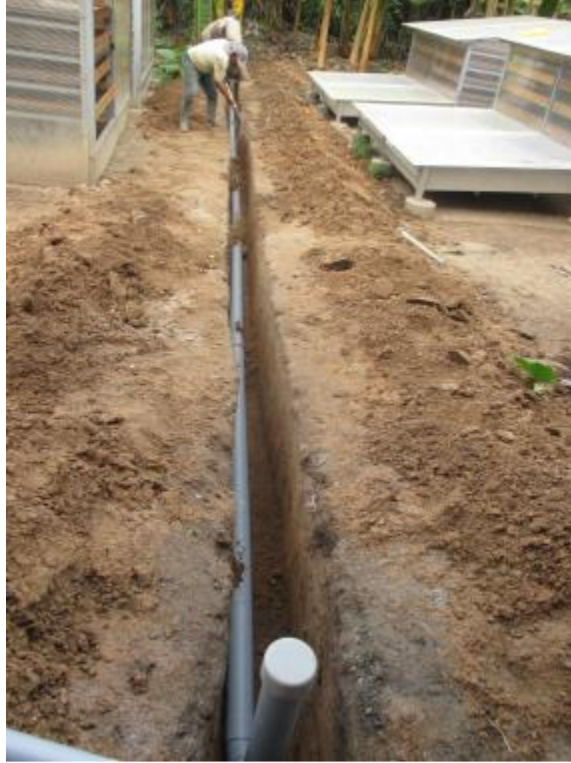
Drain piping installation.
