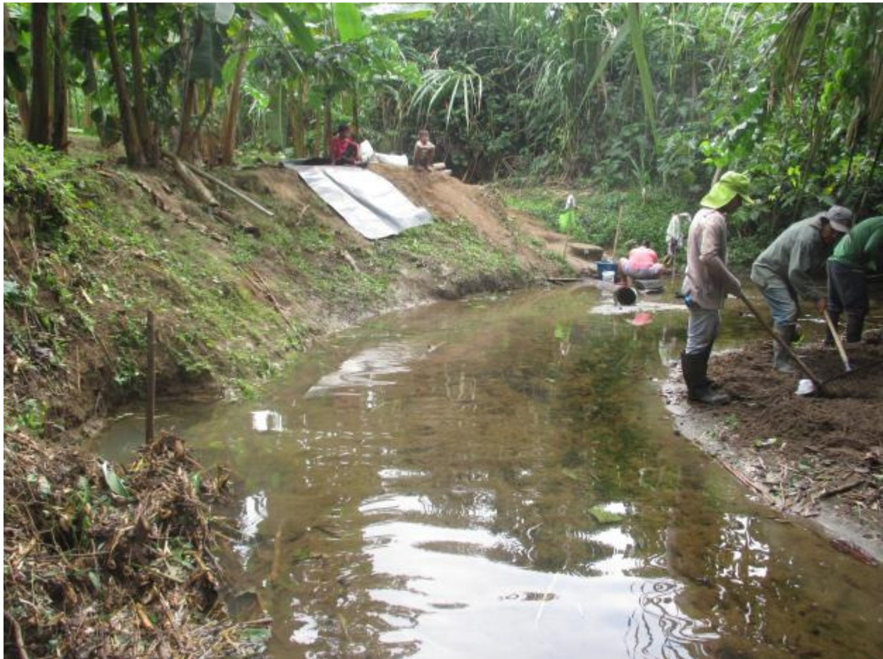
Preparing sand cement mixture across the stream from the area of stream bank erosion.
