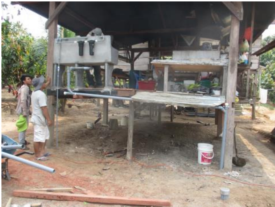
Kitchen sink with water filters and drain line.
