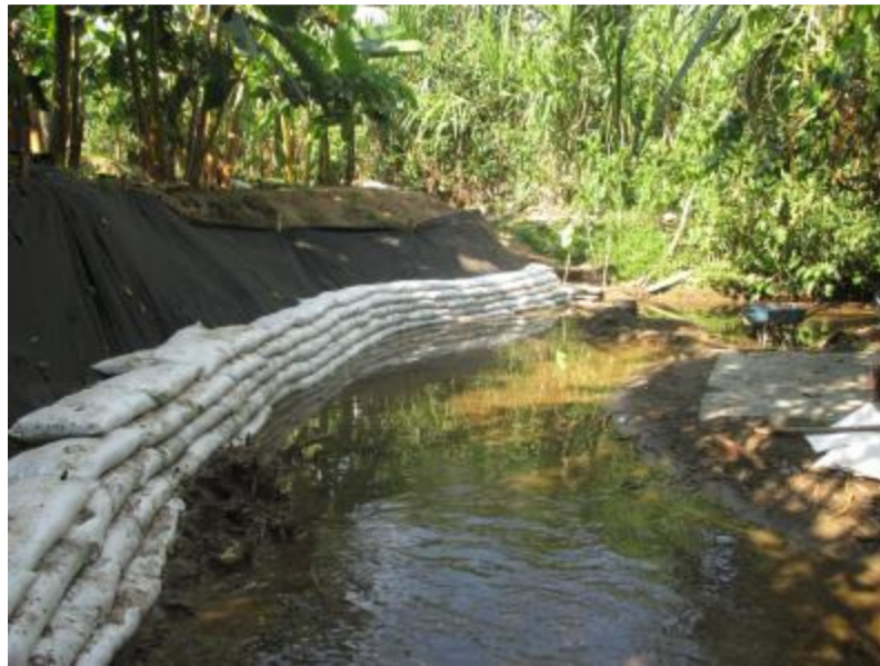
Erosion protection construction along stream bank.
