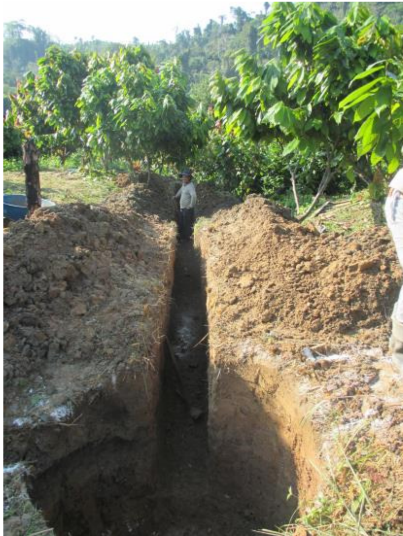
Excavation for collector tank and outlet piping.
