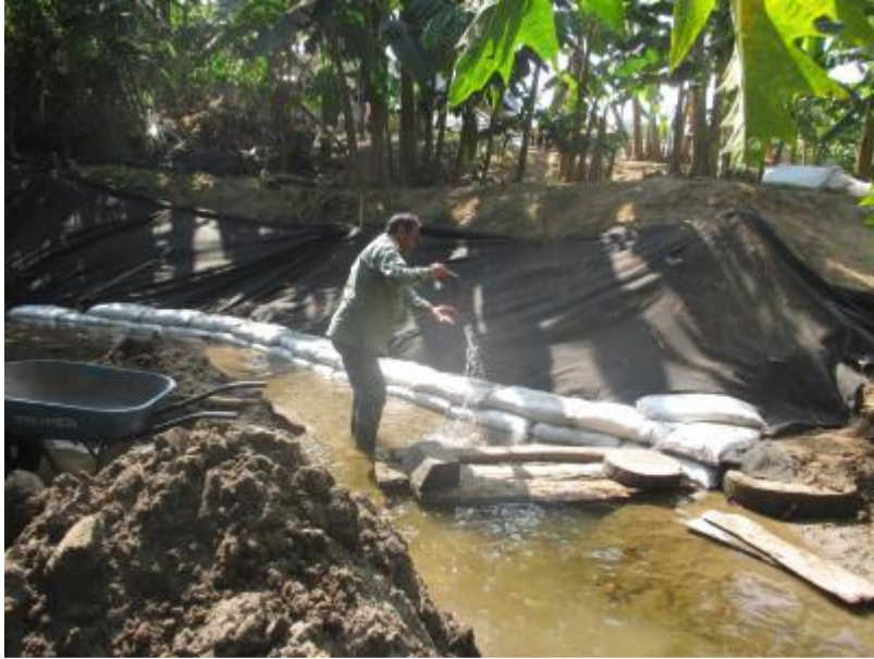
Erosion protection construction along stream bank.
