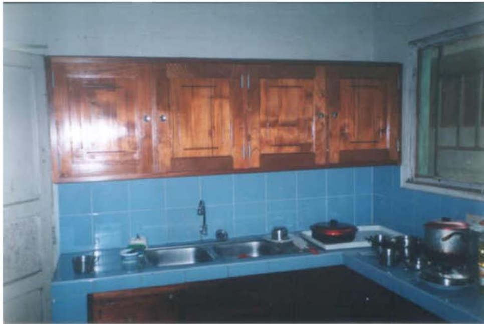
Kitchen renovation in Satipo.
