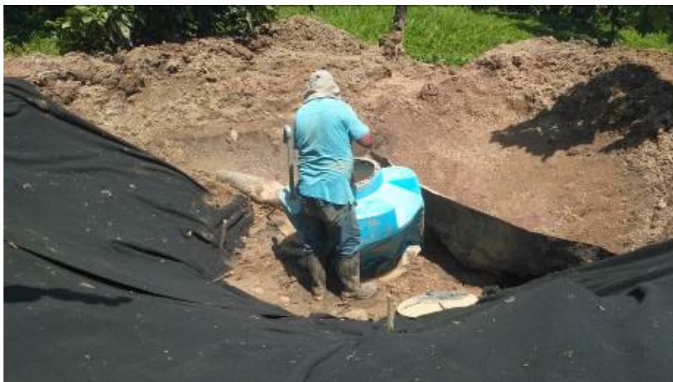
Moises working on the temporary repair for the water system tank.
