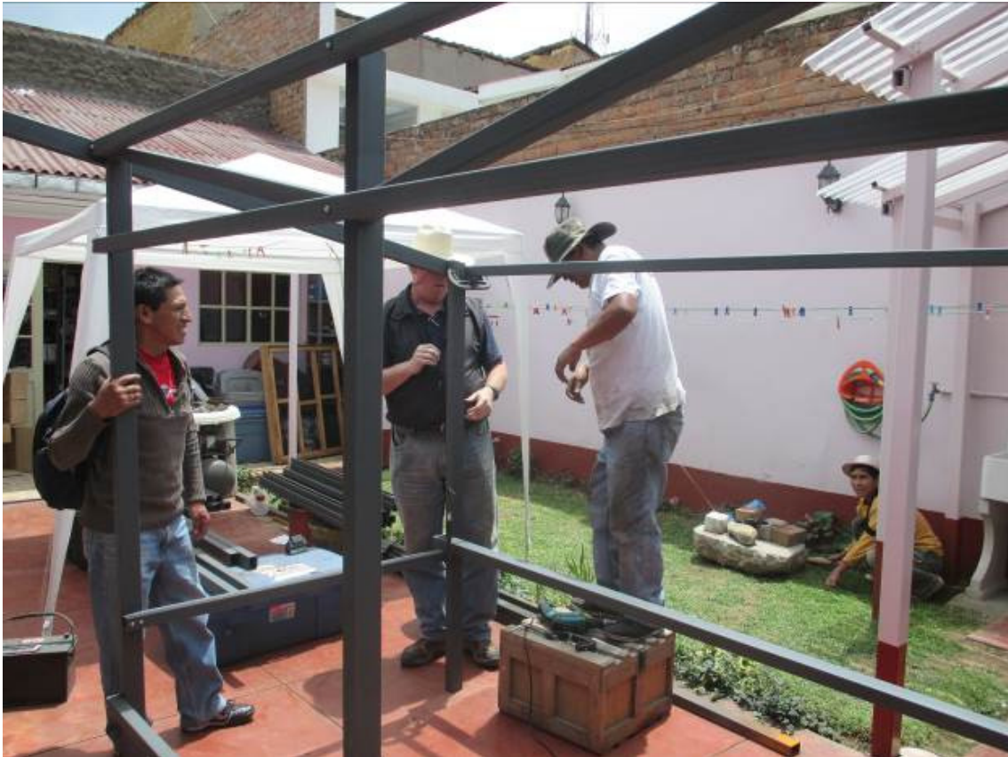
Willy, Arthur, and Moises working on the Cacao Dryer.
