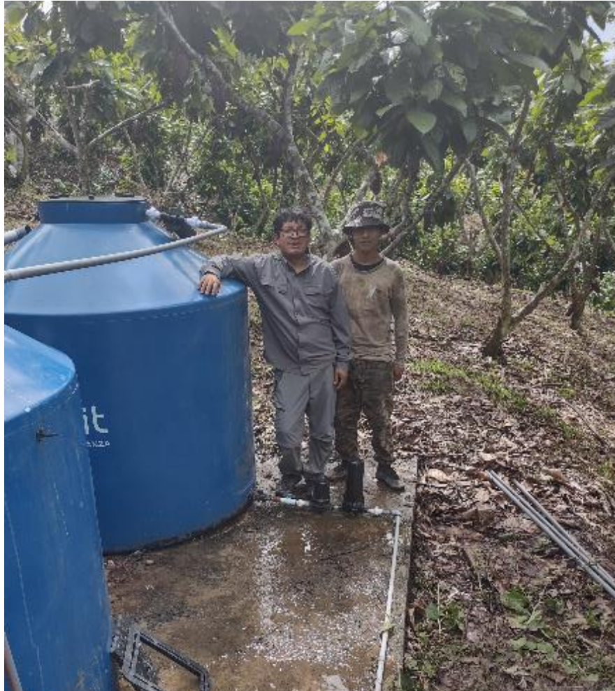
Ivan and Manuel with the water filter system.
