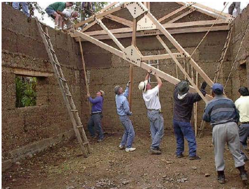
Erecting the roof structure in Ahuac
