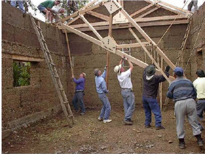
Erecting the roof structure in Ahuac
