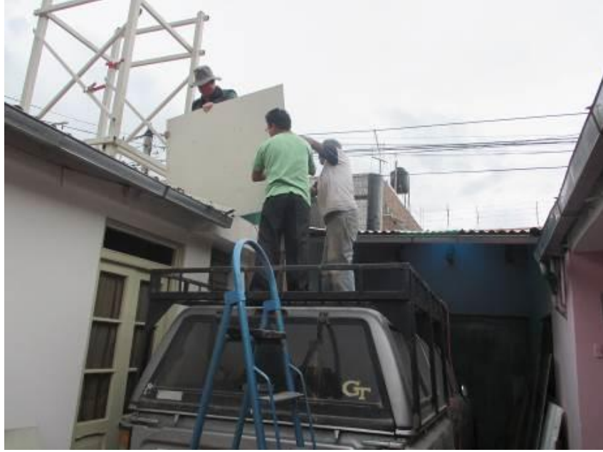
Moises, Ivan and Arthur working on the water tower
