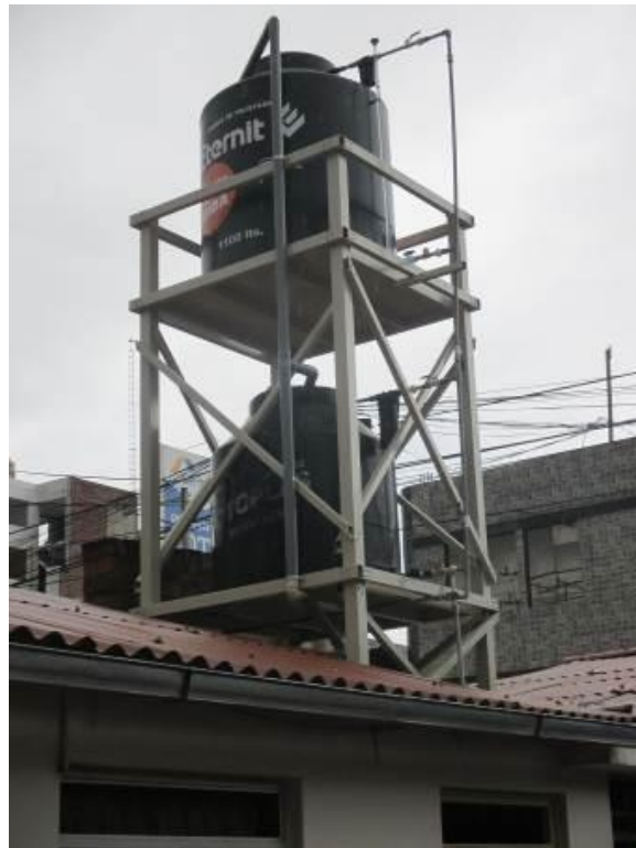
Finished water tower
