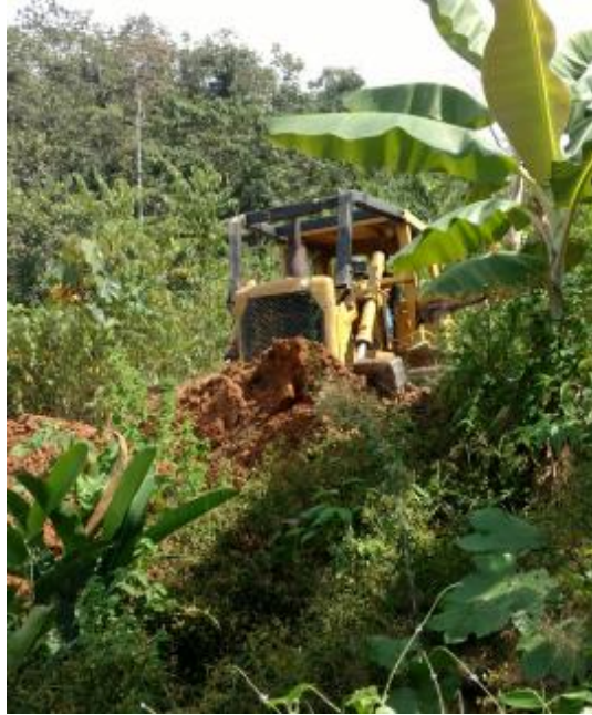
Grading the access road.
