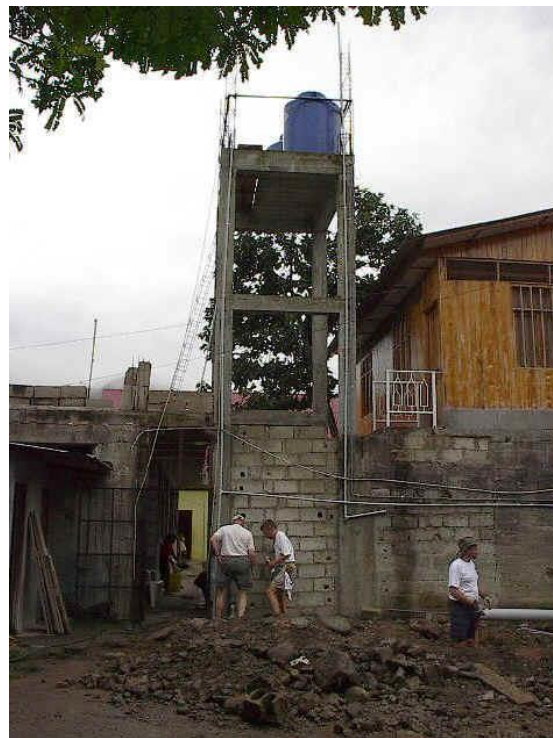
Alpharetta team installing water purification system
