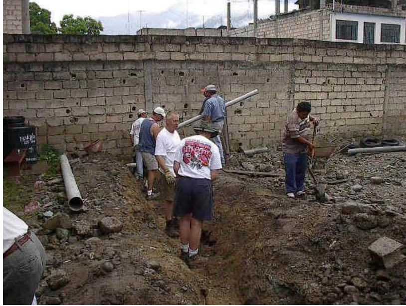
Team from Alpharetta First United Methodist Church installing sewer line at San Ramon
