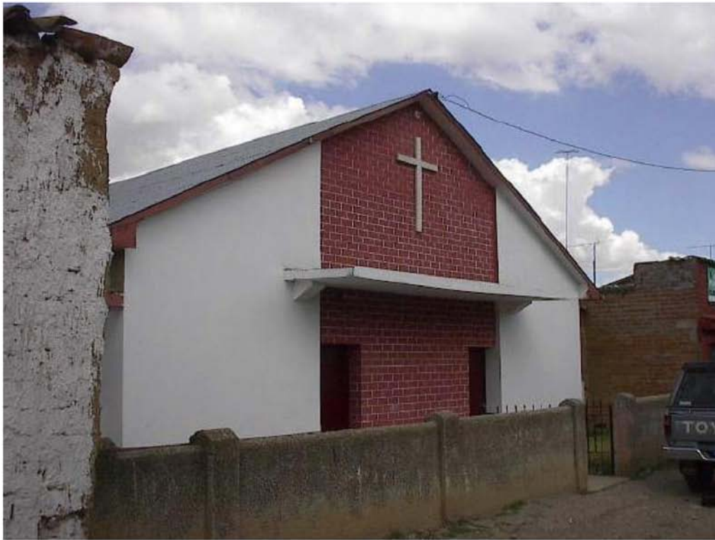
Church building in San Jeronimo
