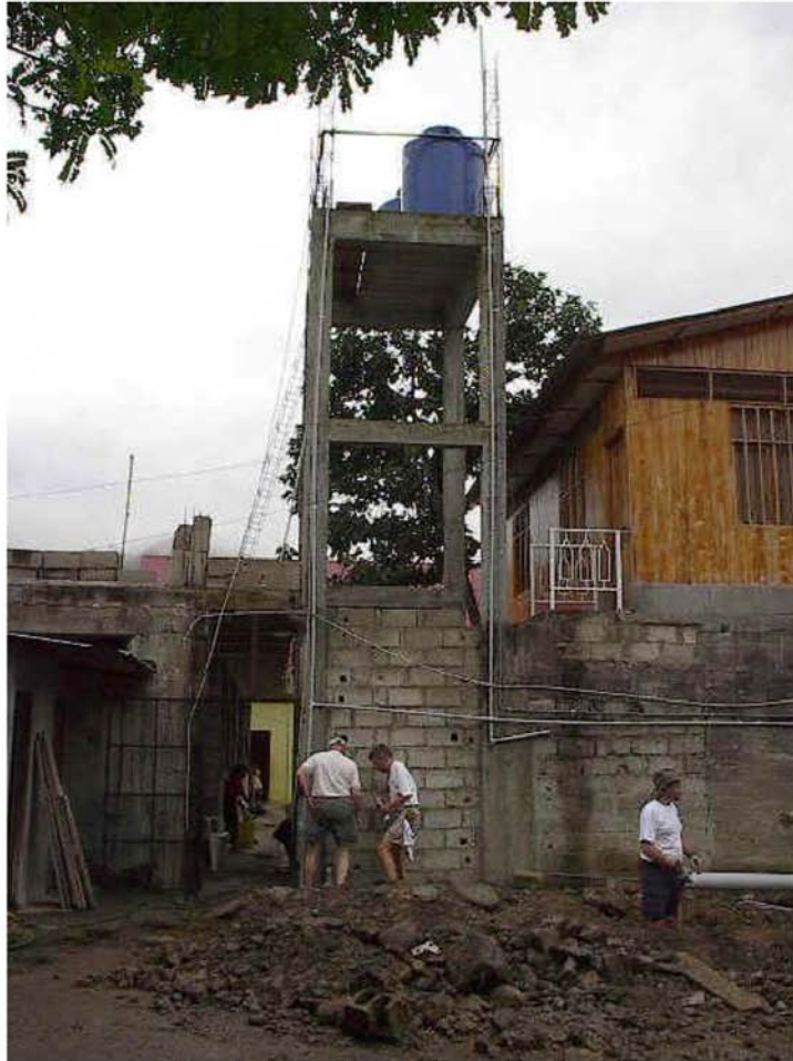
Alpharetta team installing water purification system
